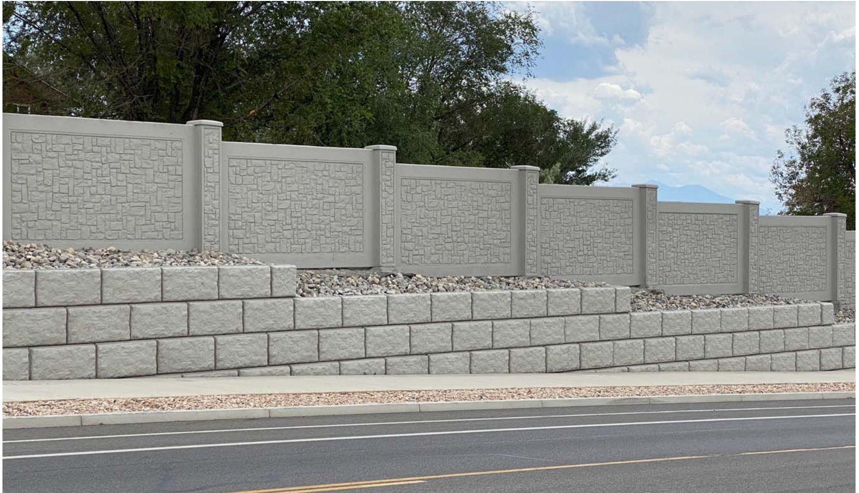
Gray Base with Retaining Wall
